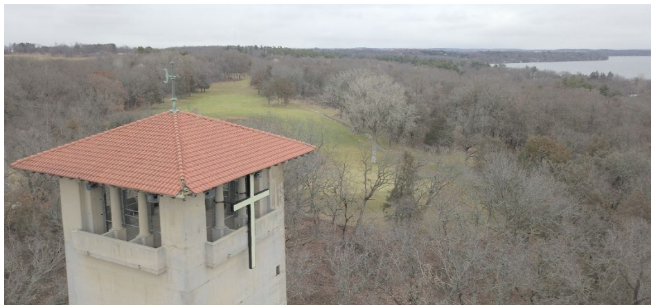
Aerial photography of the Judson Tower roof.
